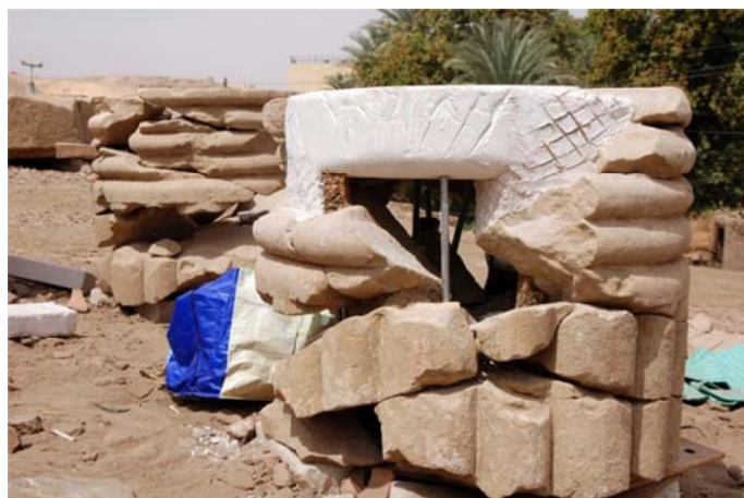
Fig. 43: Consolidation of column with stainless steel dowels (Foto: C. VON PILGRIM, SI).
