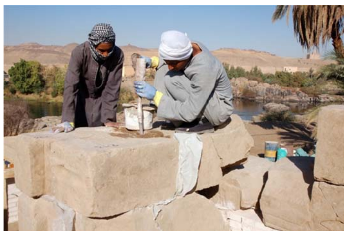
Fig. 40: Filling of joints with lime mortar (Foto: C. VON PILGRIM, SI).
